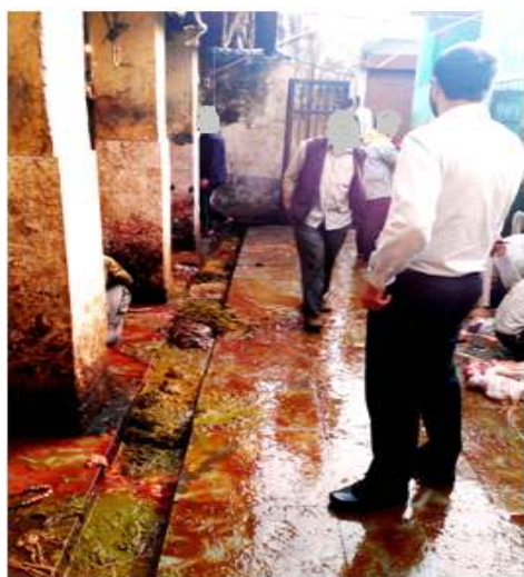
Fig. 5. Slaughter hall lacking proper drainage slope and waste disposal system
