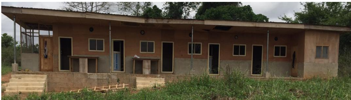
Fig. 4. Front view of the developed poultry house
